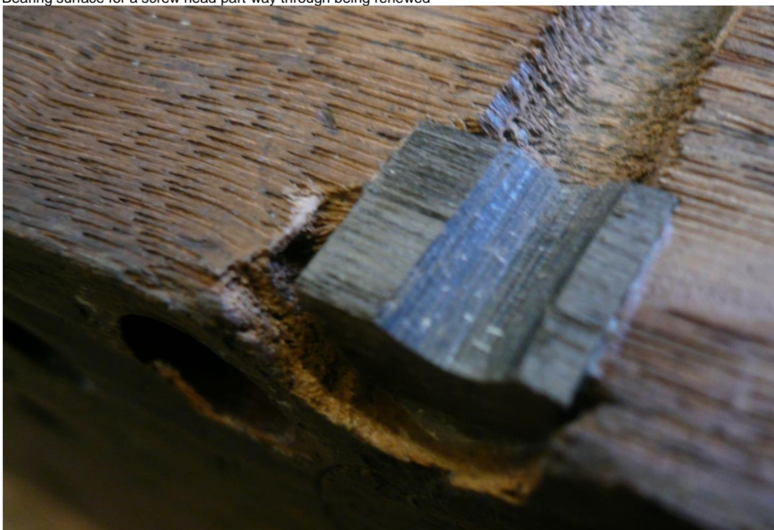
Bearing surface for a screw head part-way through being renewed
