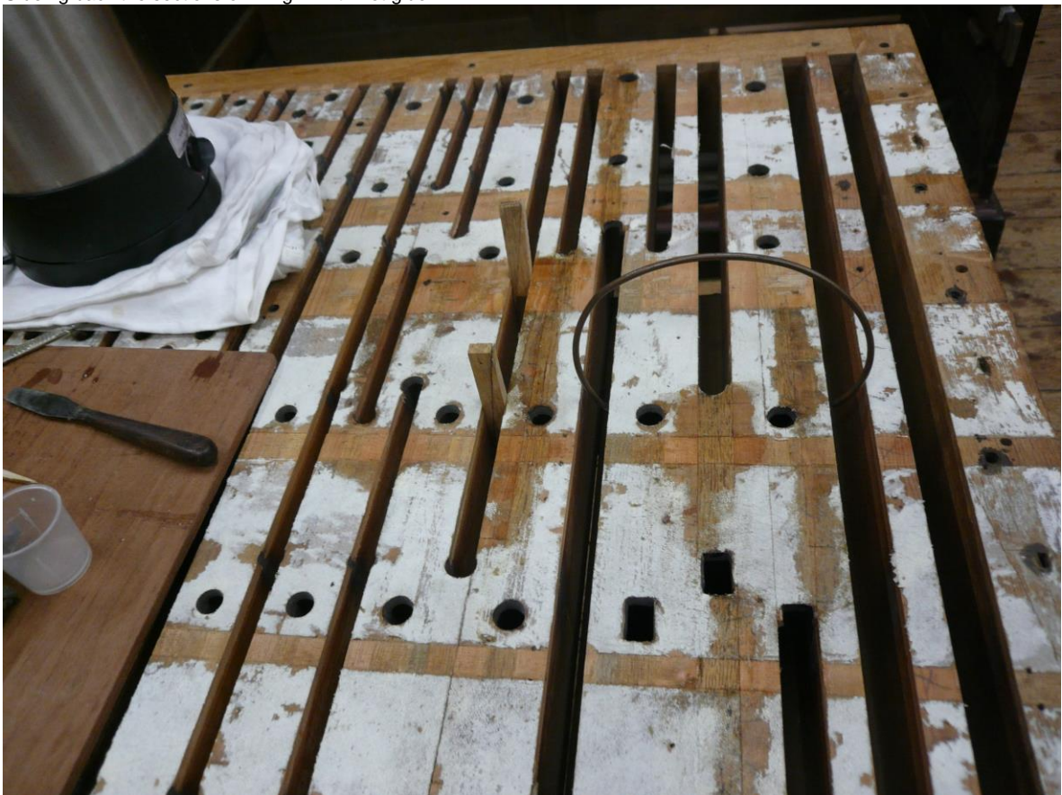
Glueing back the sections of filling-in with hot glue
