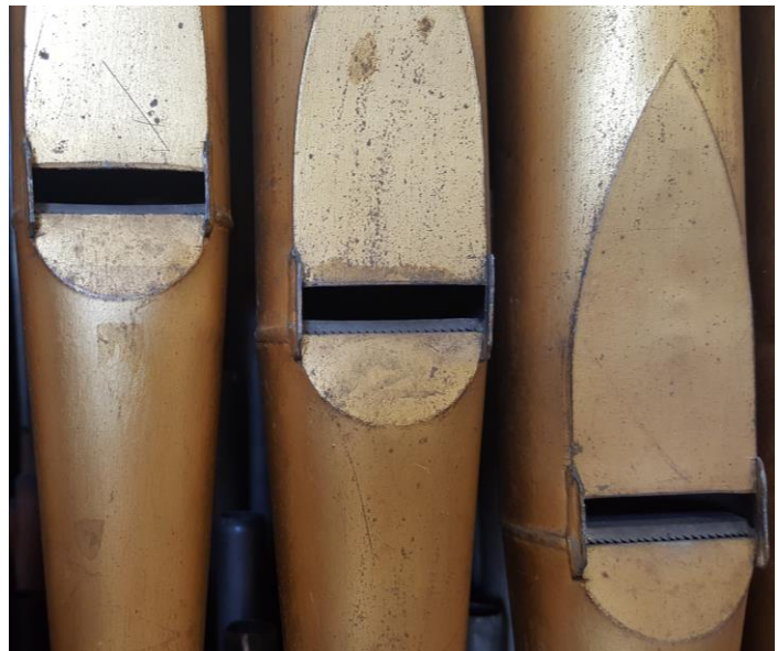
Bottom D# with a tuning flap soldered in. (note the gold leaf on the cut edge)
