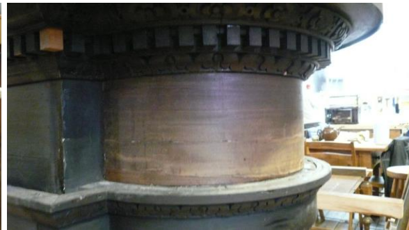
The veneer glued back in place
