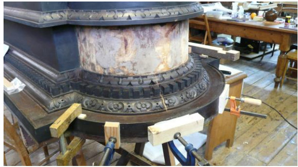
Woodworm damage filled in and surface prepared
