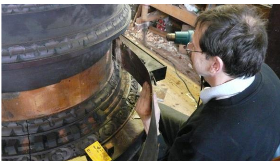
The removal of a frieze veneer
