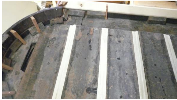
Angled shaped fixing blocks and the taped over joints
