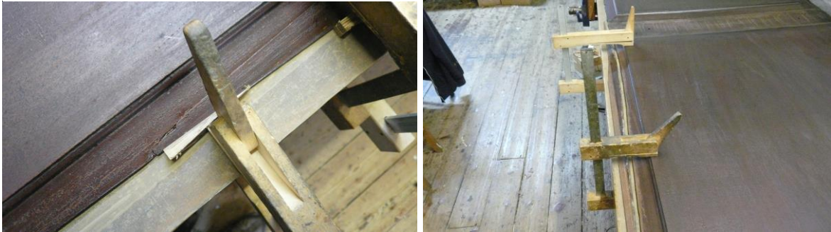
Repair of splits in edge of panels
