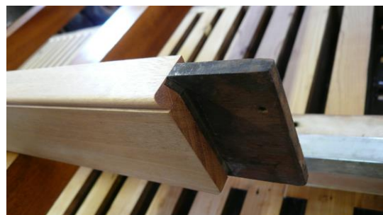
New mitres on the cocked beads to fit the old join
